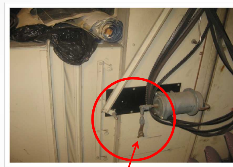
Disconnected Damper
